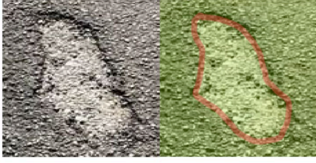
Figure. 7 The pothole ROIs are rich in road texture features (green parts), while the pothole edge features (red parts) are discarded during the texture generation process for containing strong spatial information.
