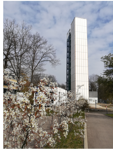
FIGURE 1. The world's first adaptive high-rise at the campus of the University of Stuttgart.
