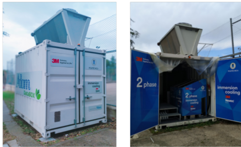
Figure 8: Two-phase immersion cooling EDC prototype.
