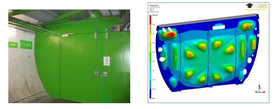
Figure 27: Door in UL46 that acts as pressure relief valve. The right part is a simulation of the deformation under a 30 mbar overpressure (deformation = 7.4 mm max.) [50].
