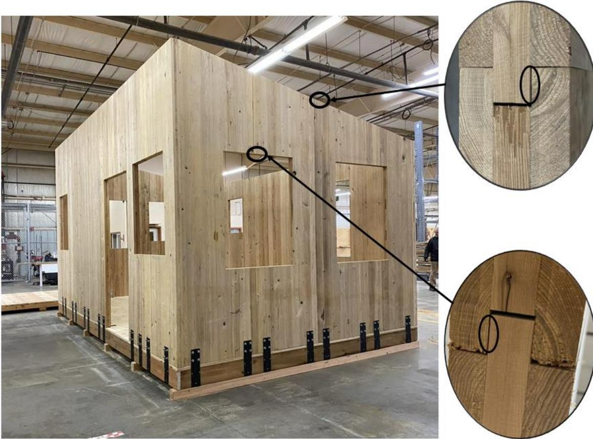
Figure 1: 22 sqm demonstration structure machined and assembled at the CRTC with thermally modified CWH CLT panels. Panels were manufactured at the Composite Materials & Engineering Center at WSU. Note that the tight 1mm of clearance is between the side faces of the t&g joint (circled) to promote panel alignment. A larger gap was intentionally designed between the end faces of the t&g joint to account for assembly tolerances.
