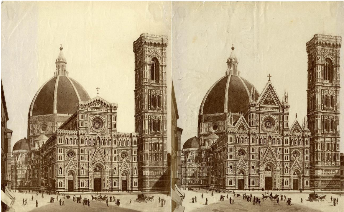
Fig. 2. Proposals for crowning the façade of the aisles submitted for consultation on January 3, 1884 (Zuffanelli and Faggia, 1887, p.16). On the left, the typical basilica crown model, on the right the tricuspid model. Niccolò Barducci, Vedute di Santa Maria del Fiore with the facciata of the De Fabris , 1876-83, Museo dell'Opera del Duomo di Firenze
