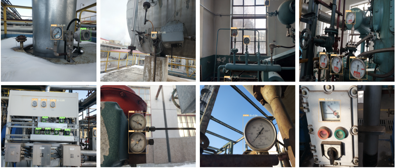
Fig.5. Qualitative results of the meter detection, where yellow bounding box means pointer meter and green bounding box means digital meter. “ID-num” is the detection confidence.
