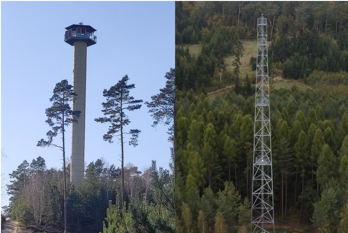
Figure 4.9: Left: Older concrete tower. At the top, there is an observation point from which the observer looked for smoke through binoculars. Currently, it is equipped with a remote camera system. Right: A newer steel tower built from the ground up with a camera system in mind, it is only accessible for servicing the cameras, without a covered observation point for a human observer.
