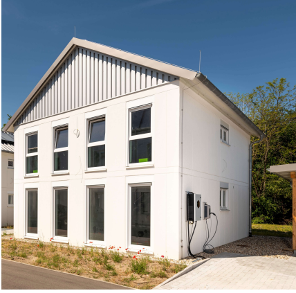
(a) Experimental building with a design similar to a single-family home
