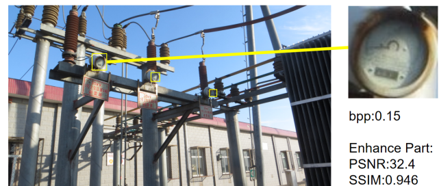
Figure 7. Visual example of the enhancement CNN model. After passing through the enhancement CNN model, the key semantic content areas of the image exhibit improved image metrics. Moreover, visually, the directions of the pointer on the panel is clearly visible.
