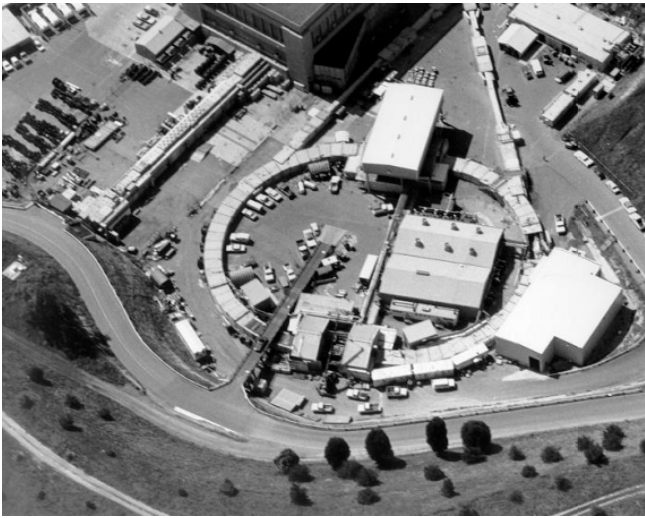
Fig. 2.1.3 The 80m SPEAR Ring in a parking lot at SLAC. The photo also shows the separate e^+ and e^- beam lines and the detector hall.
