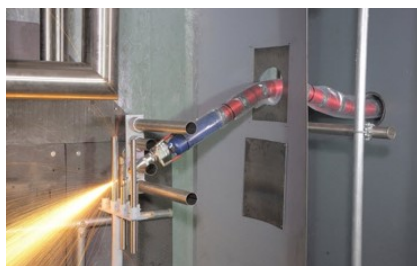
(a) LaserSnake for nuclear decommissioning
