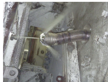
(b) Hong Kong JetSnake cleaning and inspection of TBMs
