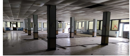
(b) Column Room
