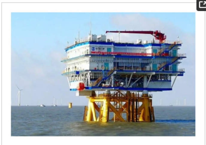
Figure 15. Offshore booster station.
