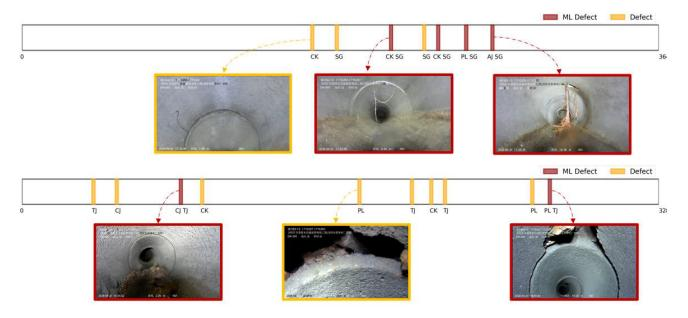
Fig. 4: Anomaly Examples of Our CCTV-Pipe Dataset. (ML: Multi-Labeled)
