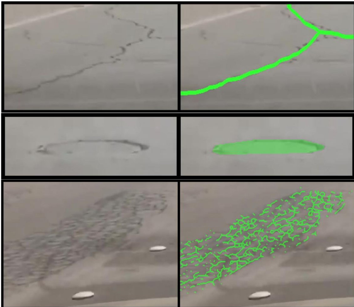
Figure 4: (left) input crop passed to the Crop Damage Segmentation module, (right) Segmented Damage (Linear crack, pothole and alligator crack from top-to-bottom) shown in Green overlaid on the input crop.
