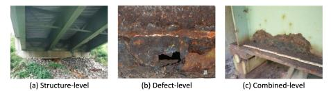
Fig. 1. Different levels of inspection images
