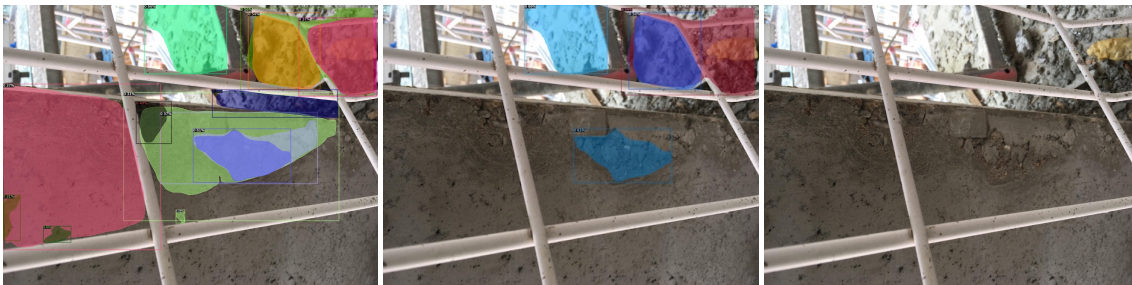
Fig. 8: Loose pebbles detected as honeycombs
