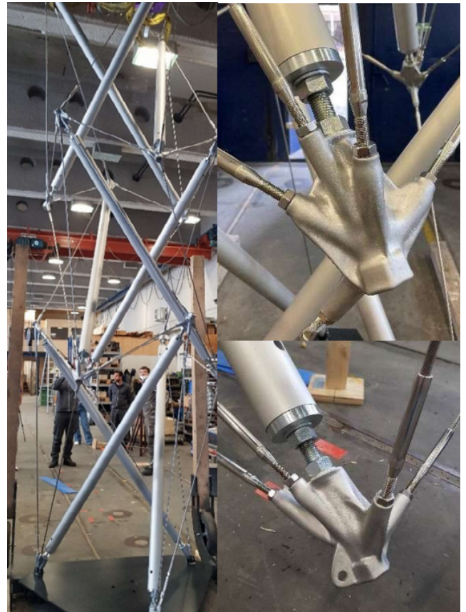
(a) The five-meter “tensegrity tower” exhibited in the Deutsches Museum of Science and Technology in Munich.
