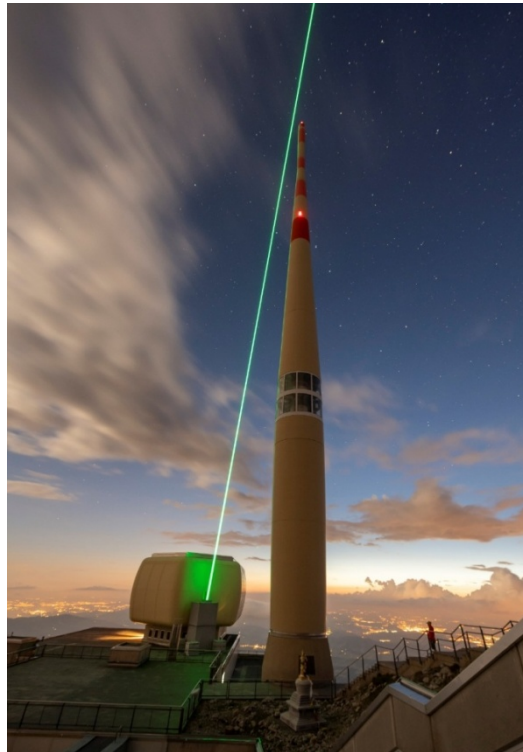
Fig. 1: Image of the 124 m high telecommunication tower of Säntis (Switzerland). Also shown is the track of the laser recorded with the second harmonic of the laser at 515 nm.
