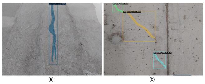
Figure 13: Examples of correctly detected (a) vertical and (b) diagonal cracks from the indoor construction site images taken using a smartphone
