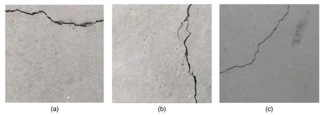
Figure 3: Different types of cracks classified in ABECIS: (a) horizontal, (b) vertical, and (c) diagonal from a horizontal perspective (source [53])
