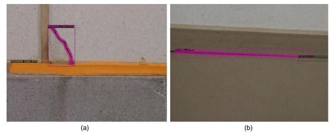
Figure 16: False positives examples from the outdoor experiment. (a) Control joint/filler between walls, identified as a horizontal crack. (b) Area between parapet wall (vertical element) and ceiling panel (horizontal element) detected as crack.
