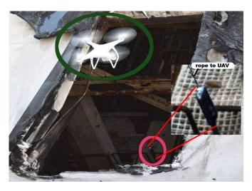
Fig. 5.  $360^{\circ}$  camera connected to the P4P with a thin rope while inspecting the hall.
