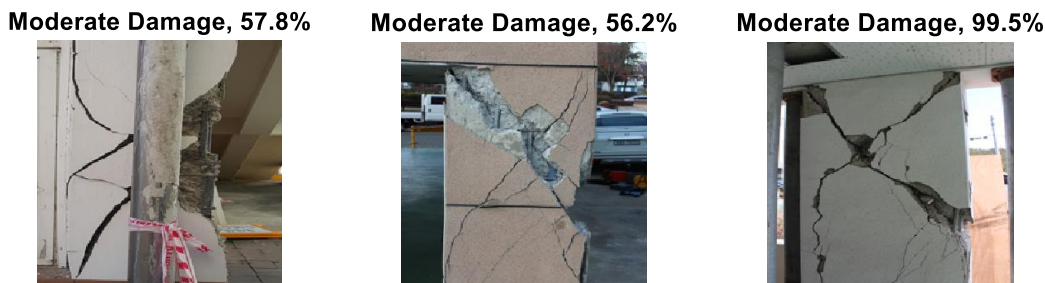
Figure 16 Unreasonable prediction of sample testing images with ground truth of “Severe Damage” as shown in Figure 8
