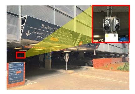
Figure 4.2: A real picture showing entrance and exit of our campus car park and a pair of LPR cameras installed side-by-side close to the ceiling of the car park ground floor.
