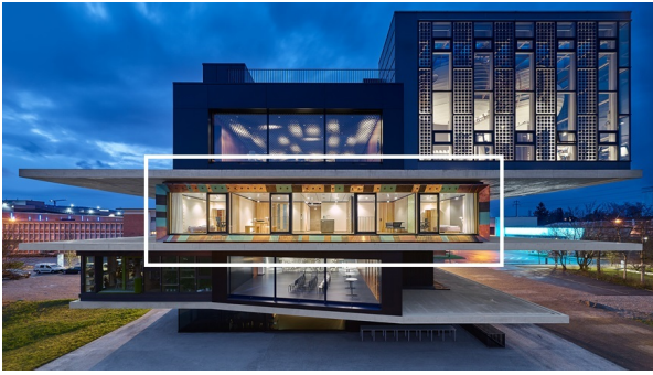
Figure 1: NEST building with the UMAR apartment unit marked in white, © Zoey Braun, Stuttgart.
