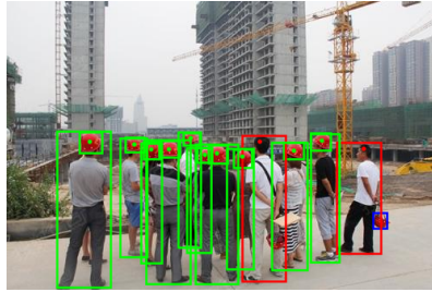
(b) failure to detect of one of the hard hats
