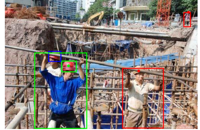
(c) failure to detect both person and hard hat due to occlusion
