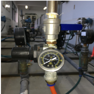
Fig. 4. Adjusting the air pressure of the pipeline
