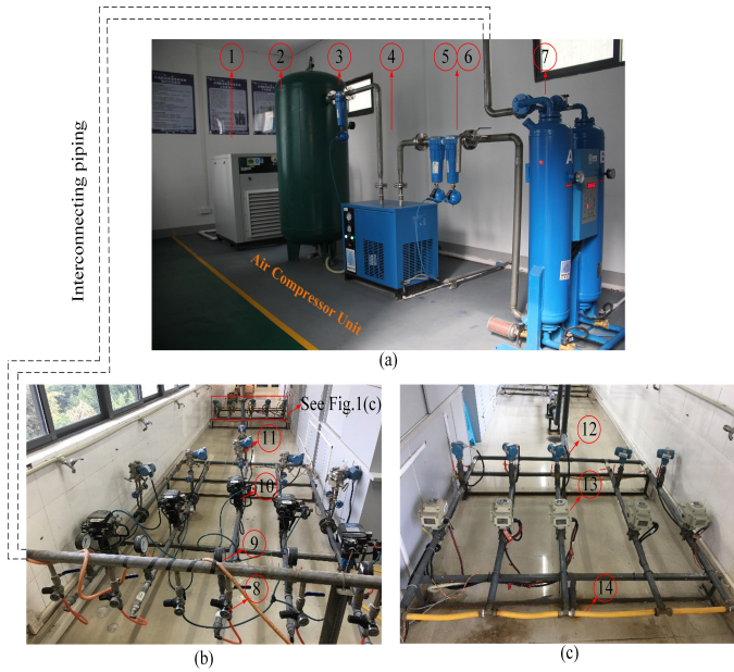
Fig. 1. Images of the gas pipeline system. (a) Air compressor units; (b) The front end of gas pipeline system; (c) The back end of gas pipeline system. Note that key components in the system are denoted with corresponding numbers (i.e., 1, screw compressor; 2, air tank; 3, water elimination filter; 4, refrigeration dryer; 5, dust removal filter; 6, oil removal filter; 7, heatless regenerative adsorption dryer (HRAD); 8, pressure regulating valve; 9, pressure gauge; 10, pneumatic control valve; 11, different pressure orifice flowmeter; 12, pressure transmitter; 13, electric control valve; 14, gas discharge tube).
