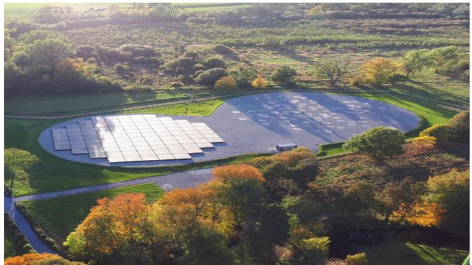
Fig. 1. I-LOFAR station located in Birr, Co.Offaly, Ireland. This an international station consisting of 96 Low band antennas (right) operating between 10-90MHz and 96 High band antennas (left) operating between 110-250MHz.
