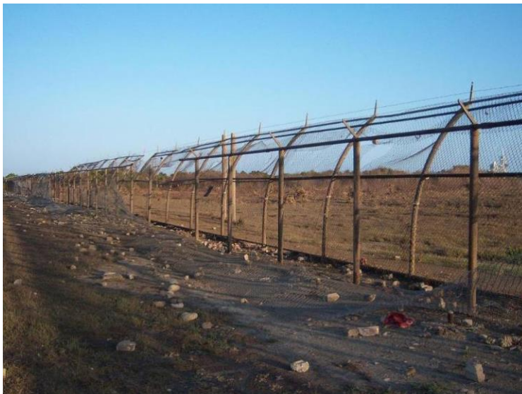
Figure 1. Thousands of bricks blown loose by the STS-124 launch, destroying parts of the pad perimeter fence.
