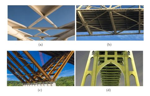
Figure 2: The typical steel bridges structure: (a) cross shape, (b) K-Shape, (c) L-Shape, (d) and combination of shapes
