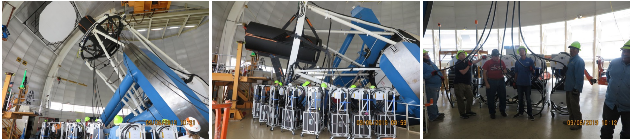
Figure 5. The fiber cables and slits were stored on their shipping carts during the focal plane installation and handled by an expert team of NOIRlab engineers during cable routing.
