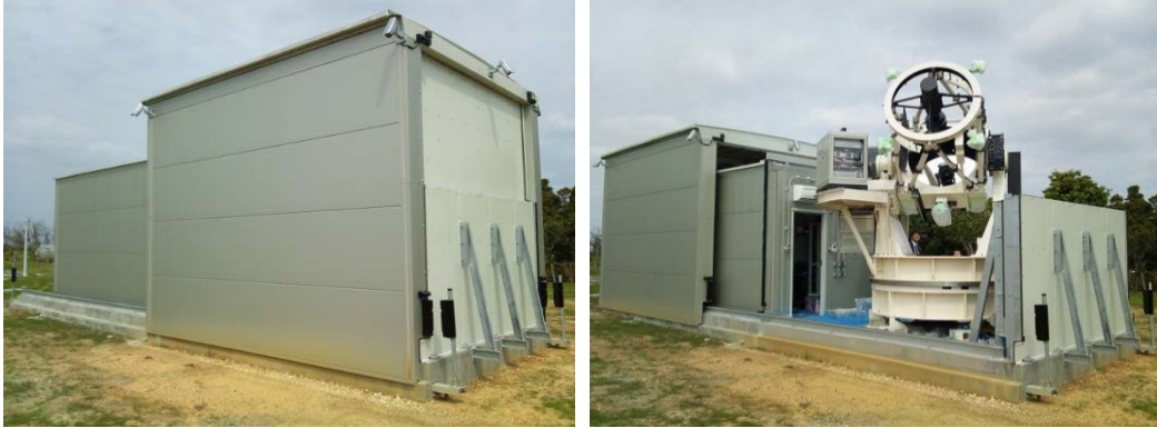
Fig. 8.26. Compact and remotely-controlled 1-m OGS in Okinawa (Japan) built by NICT.
