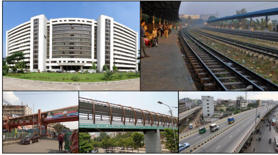
(a) Building, railline, concrete overbridge, steel overbridge, flyover
