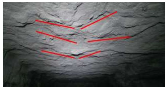
Figure 3. Roof beams on the mine roof
