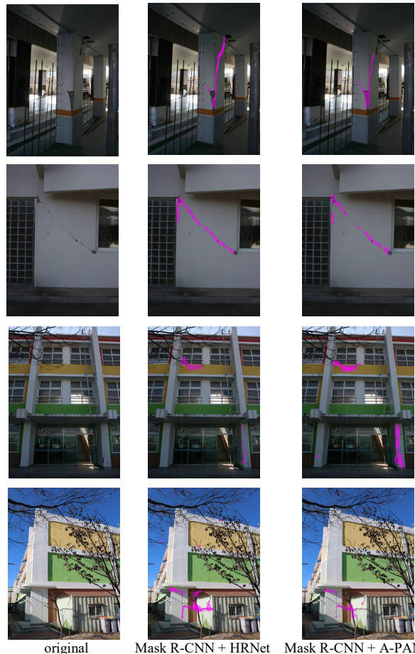
Fig. 11. Prediction of Mask R-CNN with Attention PANet and HRNet for 2017 Pohang earthquake images [32].
