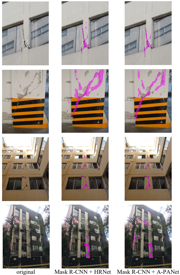
Fig. 10. Prediction of Mask R-CNN with Attention PANet and HRNet for 2017 Mexico City earthquake images [33].
