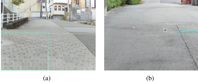
Fig. 13. Illustration of domain shift complications (a) poor generalization to new pavement types (b) dead leaves are detected as damages, showing that different seasonal features may impact generalization.
