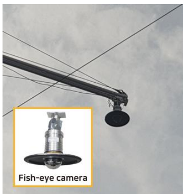
(a) Fish-eye camera Installed 15m high
