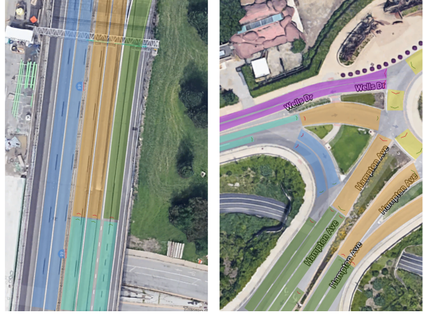
Figure 3: An illustration of lane sets under two different situations overlapping on a satellite map, the left is on highway exit, the right is a complicated lane topology near a roundabout, the red and green arrows represent entrances and exits of those lanes
