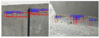
Fig. 1. Conflict between poor *mean Average Precision* (mAP) score and fine visual performance in crack detection. Demo images and their AP scores of the general objects (left) and cracks (right) are presented. According to the visual performance, the crack detector should not be such low scored (33.2).
