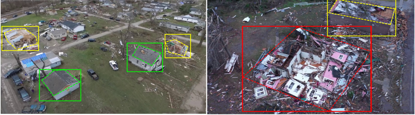
Figure 2. Visualization of our ISBDA dataset. The green, yellow and red polygons denote damages in Slight, Severe and Debris levels, respectively. The rectangles composed of solid lines represent damaged building bounding boxes. The polygons with dotted lines represent segmentation masks of damaged parts.
