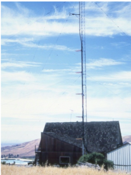
Fig. 15. House close to a radio broadcasting tower in San Jose - CA (photo by Richard A. Tell). The EMF field measured in the proximity of the house was higher than 61.4 [V/m].
