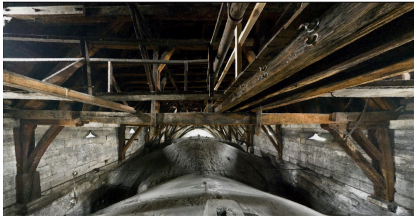
Figure 5: The charpente of the choir; the top of the guttering wall was, before \sim 1220 , at the level of the corbels supporting the wall pieces and braces beneath the fermes (extracted from Tallon [2019] ).
