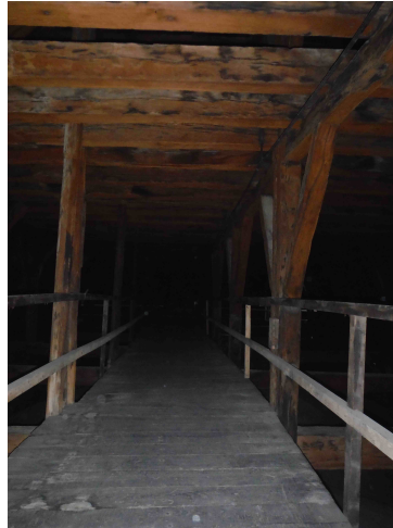
Figure 9: The catwalk; the suspente is the vertical tie on the left, while the poignon the one on the right, with its aisseliers (by the author).
