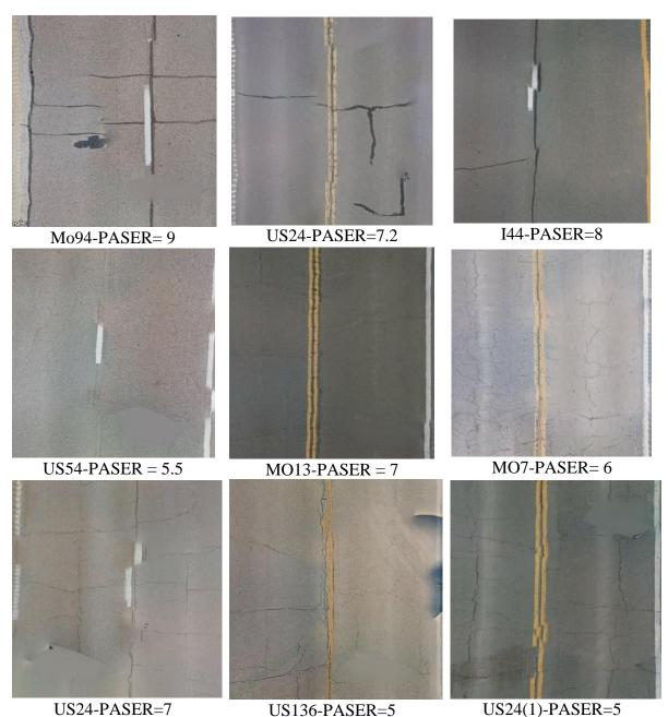
Figure 5. Example of inconsistency in PASER rating among the investigated sections
