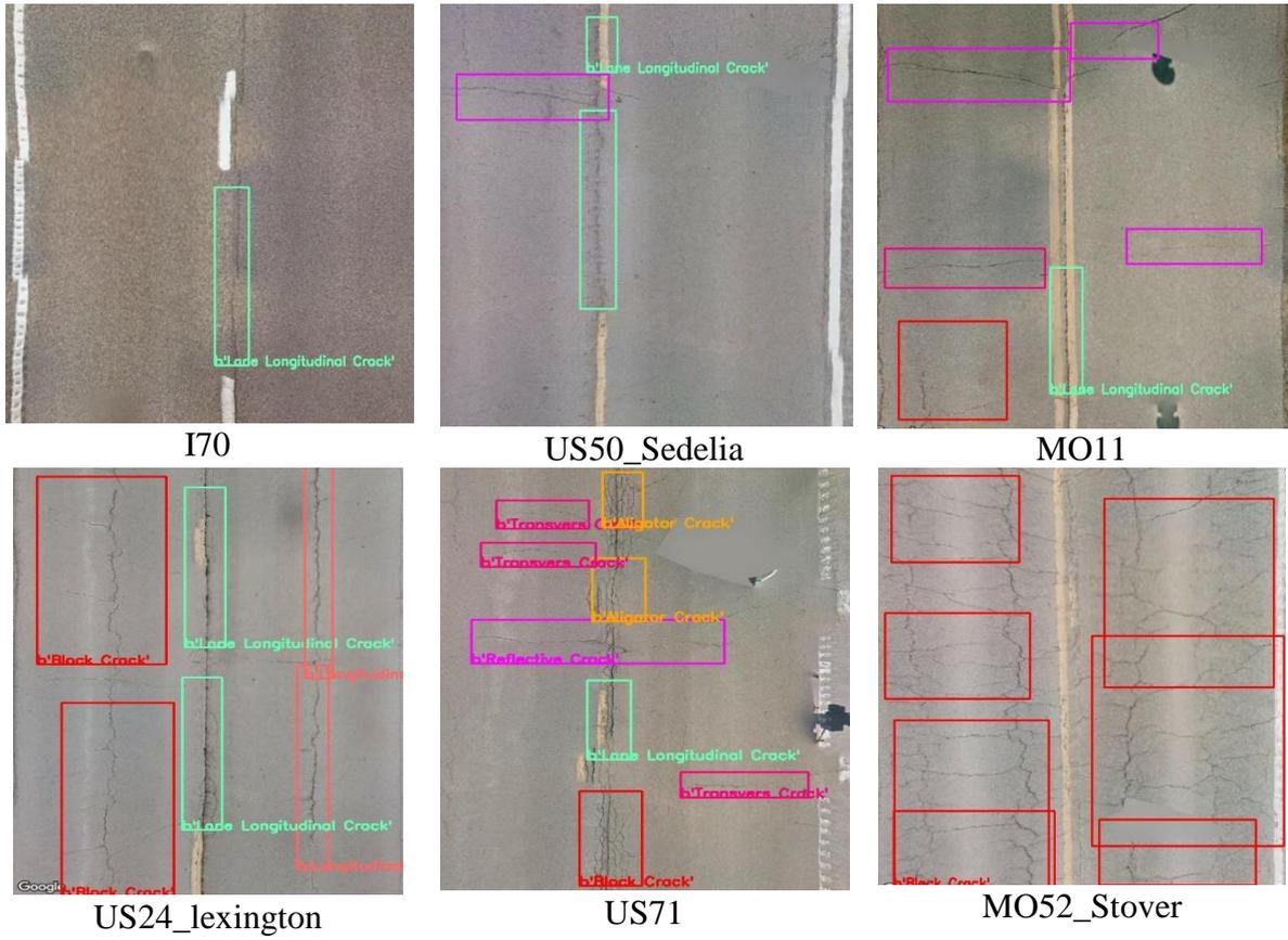
**Figure 21.** Pavement condition, a) I70 (good condition), b) US50 , c) MO11, d) US24, e)US71 and f) MO52 (dense-block cracks).
