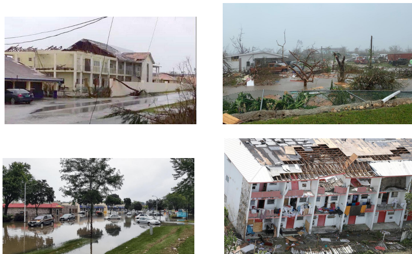
Figure 6. Mild damage images identified by the automatic system
