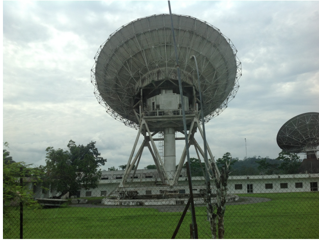
Figure 5. Decommissioned 32 meters large Satellite Earth Station antennas in Gabon.
