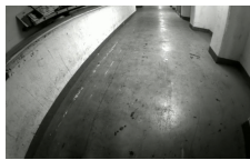
Basement (610 frames, 2978 keypoints)
