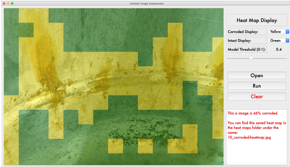
Figure 8: Visualization of an image identified as corroded using the GUI. The corroded areas are highlighted using yellow color and intact areas using green color.
