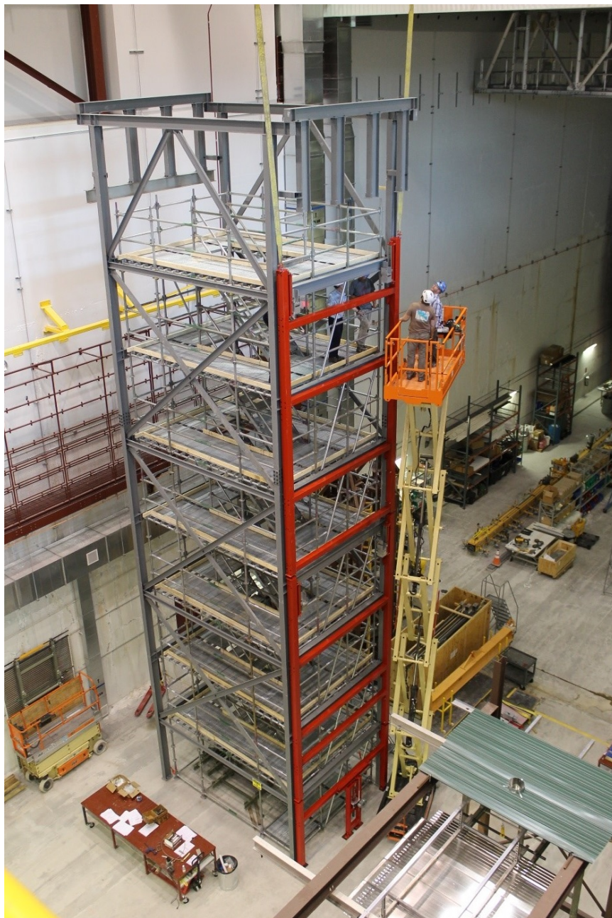
Figure 4.6: Phase 1 anode plane assembly (APA) installation frame (in red) being installed on the APA assembly tower at Ash River. In the foreground is the ProtoDUNE-SP trial assembly structure.
