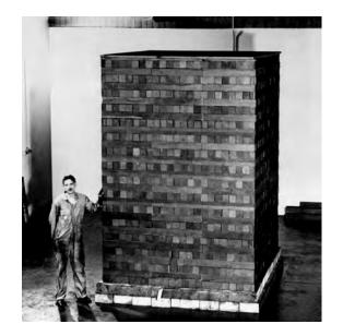
**Fig. 2.** Likely an early exponential pile. If the man is about five feet tall, this was probably an 8 by 8 by 11-foot exponential pile. *Source: https://www.atomicheritage.org/history/chicago-pile-1*
