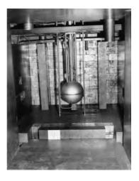
**Fig. 5.** The Los Alamos LOPO reactor. Source Courtesy Atomic Heritage Foundation; https://www.atomicheritage.org/history/water-boiler-reactor
