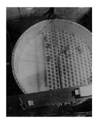
Fig 8. Kurt Diebner's paraffin-honeycomb G-I pile. Image courtesy Mark Walker.
